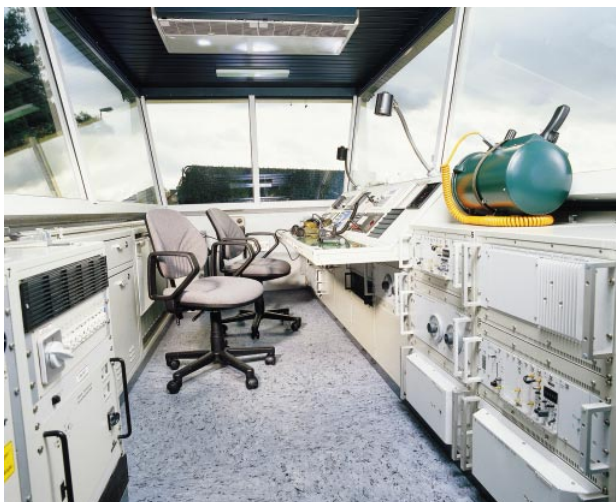
Inner view of MATC tower (Photo 40783-3)
